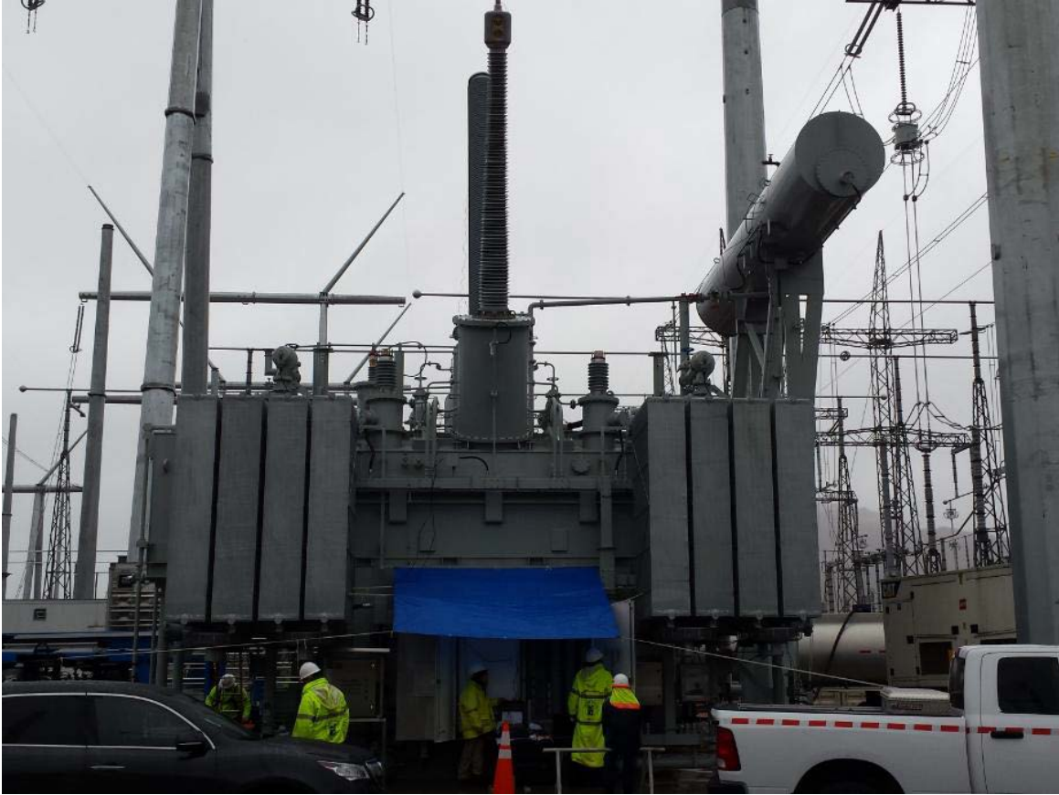
Figure 12: Picture showing the testing under energized lines and rainy condition
